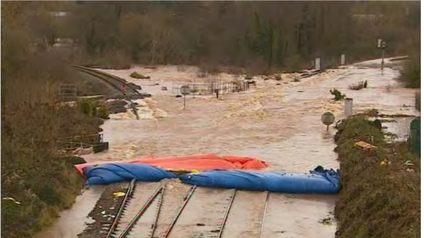
Flooding by the River Exe at Cowley Bridge Junction outside Exeter. The line to the left is the Barnstaple branch whilst the inflatable booms are an effort to keep the worst of the water out of the signalling equipment..
