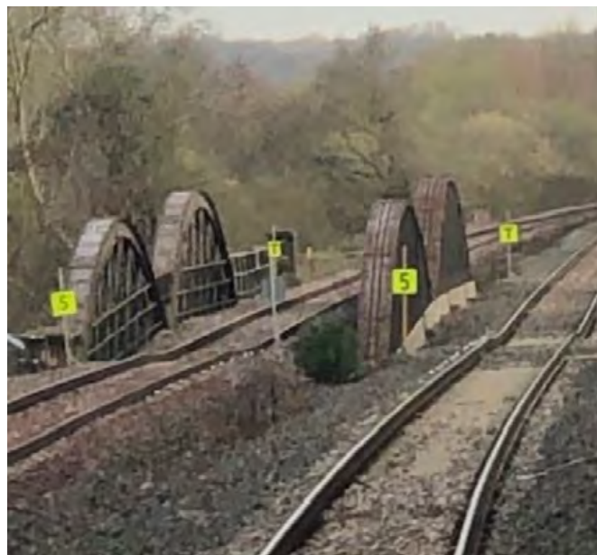
A track level view just after the closure showing how far the bridge and track had dropped.
