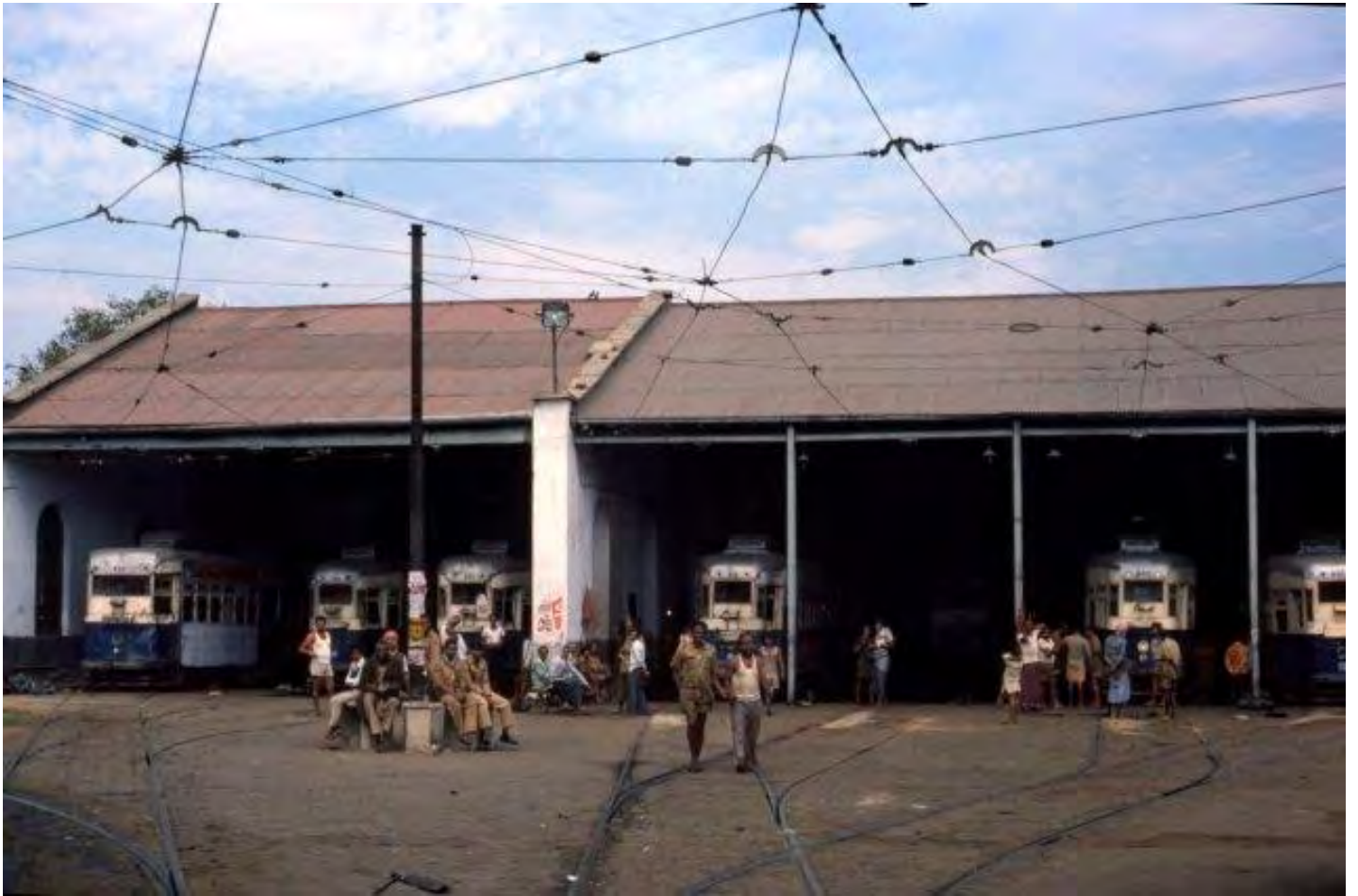
Kidderpore Tram Depot – note the spider's web of overhead lines!
