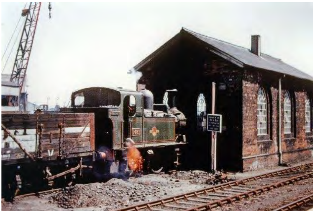
The fire is thrown out of 1421 as it stands outside Marlow shed during the midday break on 29th June 1962. The coal wagon would be a perfect model. .
