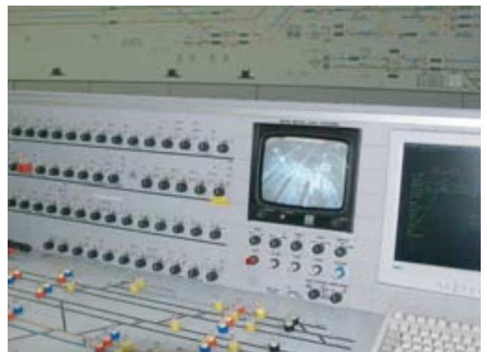
BELOW: A close up of work station 3 showing the CCTV monitor and controls for the Mitre Bridge Level Crossing. The bank of switches to the left of it are to control points individually. The entrance-exit route setting buttons can be seen on the main panel below.
