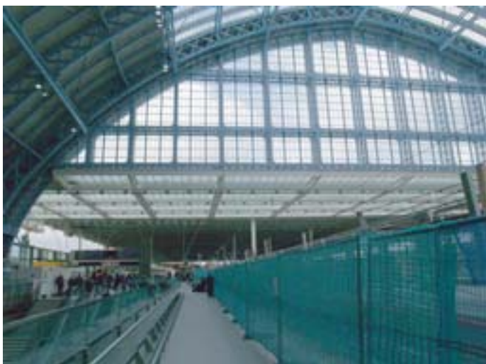
The north end of St Pancras showing the interface between the old and new trainsheds.
