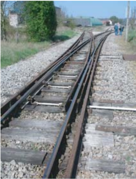
These two photographs show the complications of mixed standard and metre gauge tracks on the C F Baie de Somme. Note that here there are separate rails for each gauge.
