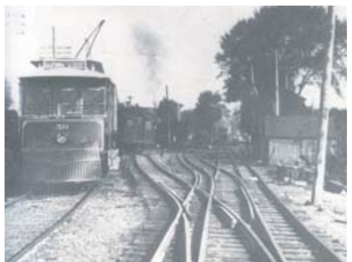
Triple gauge pointwork on the Cincinnati Georgetown & Portsmouth. The interurban car is 5' 2½" gauge.
