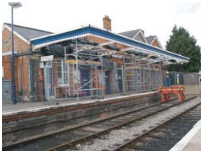
Bourne End Station surrounded by scaffolding on 30th July.
