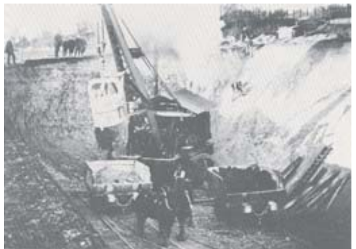
The Joint Line was built sufficiently late to take advantage of mechanised construction techniques. Here a steam shovel works in the cutting on the Saunderton cutoff.
