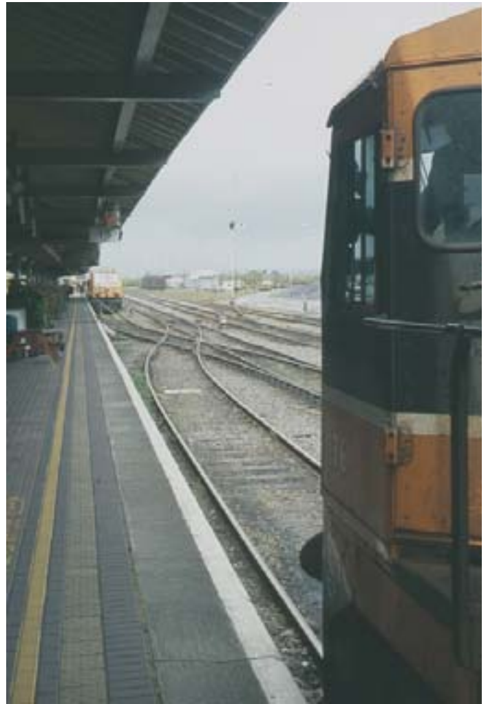
Looking east from the former Dublin platform (F) showing the half-scissors crossing at mid platform. A Dublin to Cork train does business at the far end (E) whilst an Engineer's train waits in the foreground.
