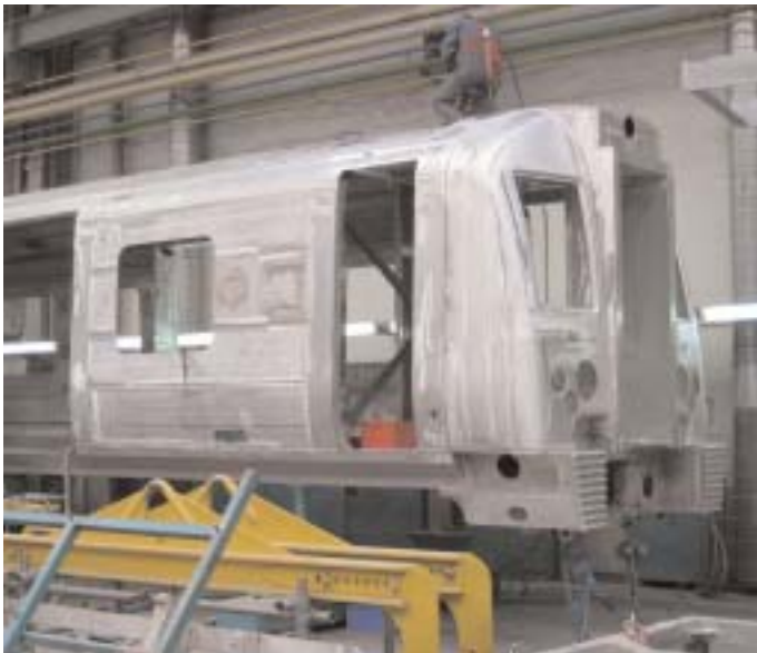
Below: Not quite Budd, but it is aluminium, after all. 350 front end - note the welder on the roof.
