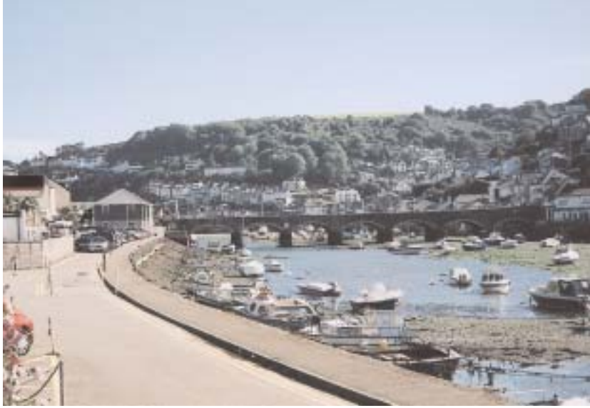
Looe road bridge between West Looe (right) and East Looe (left). In the foreground the trackbed of the line extending from the present station to the site of the former GWR terminus just beyond the parked cars. Sep 04
