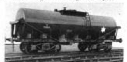
40-ton Bogie Tank Wagon for liquids
