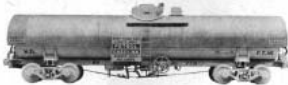
Bogie Petrol Tank Wagon for Nyasaland Railways, 2' 6" gauge.
